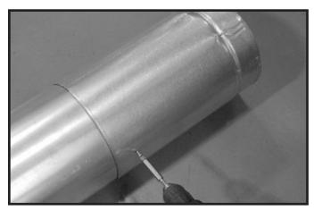
Figure 10.4 Screws into Slip Section
